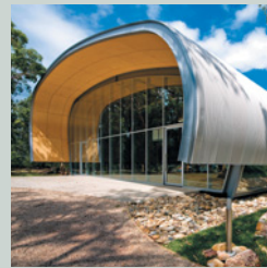
Roof and walls: Dune®
